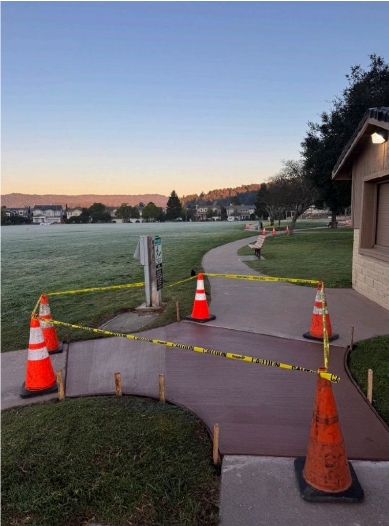
Repairs at Skypark
